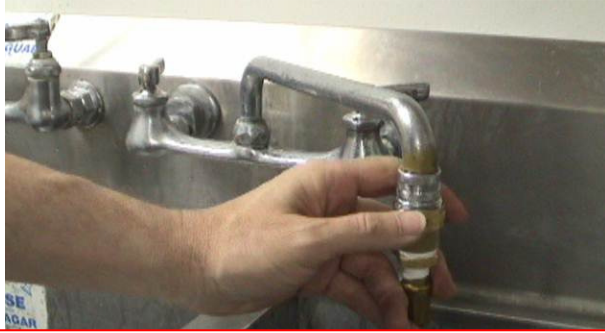
Connect the Auto-Fill Water Supply Hose to a faucet and turn on the water
